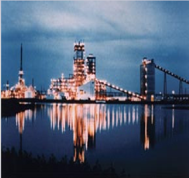
A 250-megawatt IGCC power plant near Lakeland, Fla., constructed as part of the U.S. Department of Energy's Clean Coal Technology Program. DOE photo.
