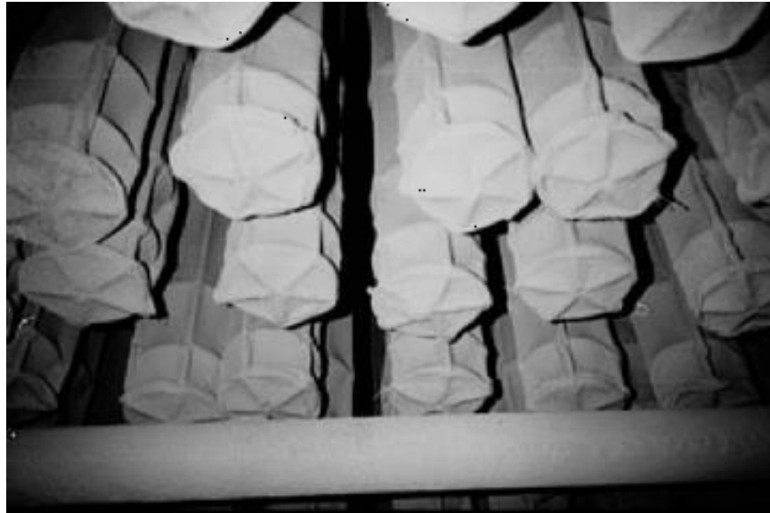
Figure 4-2. View of the bottoms of pulse jet bags (note flex around inner cages)
