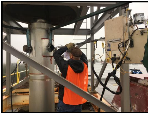
Stack Emission Sampling
