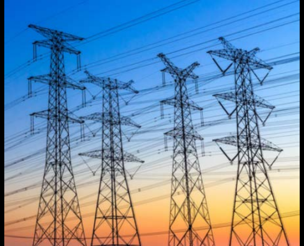
Average 527 kWh - power for 400+ homes
