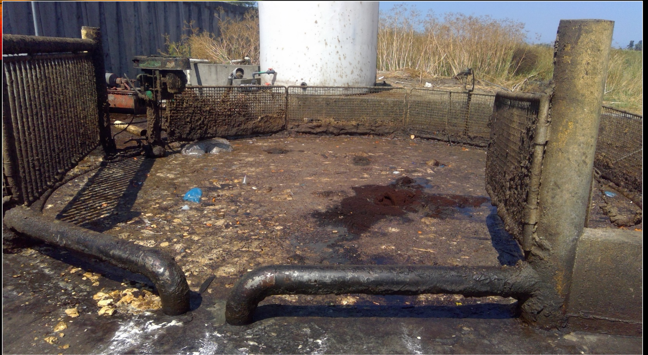
Off-site waste (e.g., food processing waste, restaurant grease) up to 30% of biomass
