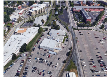
Viant Medical Facility
