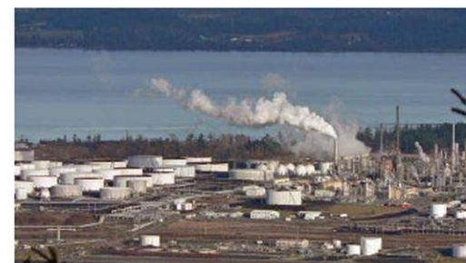
The Shell Puget Sound Refinery on the south end of March Point. Padilla Bay is in the background. (Photo: Shell)
