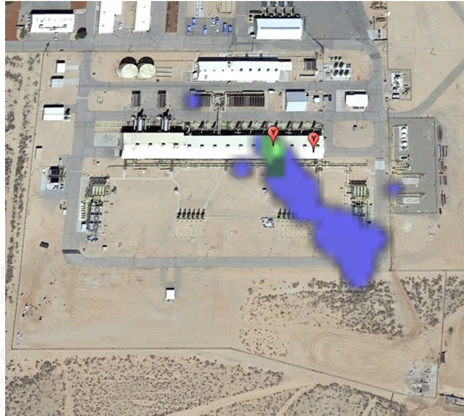
• Leaking natural gas compressor station
