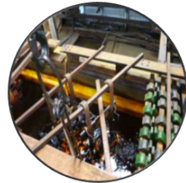
Metal Processing Facilities
