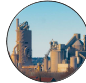
Cement Batch Plants
