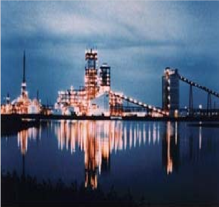
A 250-megawatt IGCC power plant near Lakeland, Fla., constructed as part of the U.S. Department of Energy's Clean Coal Technology Program. DOE photo.
